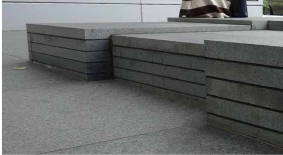
Granite Retaining Wall
